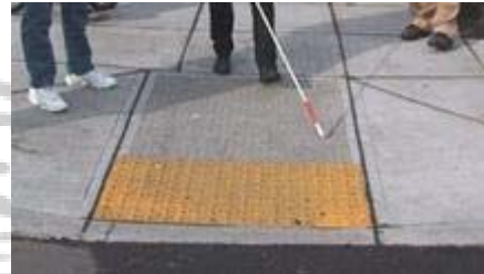
Fig. 4-1: Truncated domes help the visually impaired determine where the sidewalk meets the street.
