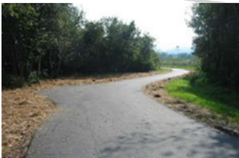
Fig. 7-2: A section of the completed first phase of Brevard's MUP System.
