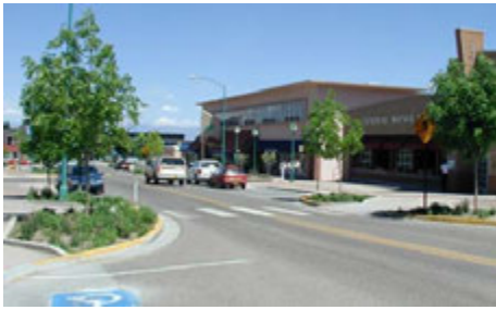
Fig. 6-1: Bulb-outs (left) and raised crosswalks (right) can be used together or separately to increase visibility of pedestrians to drivers.
